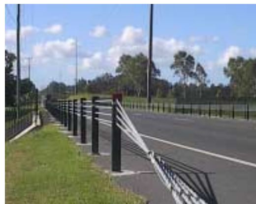
Picture: Wire Rope Safety System.
