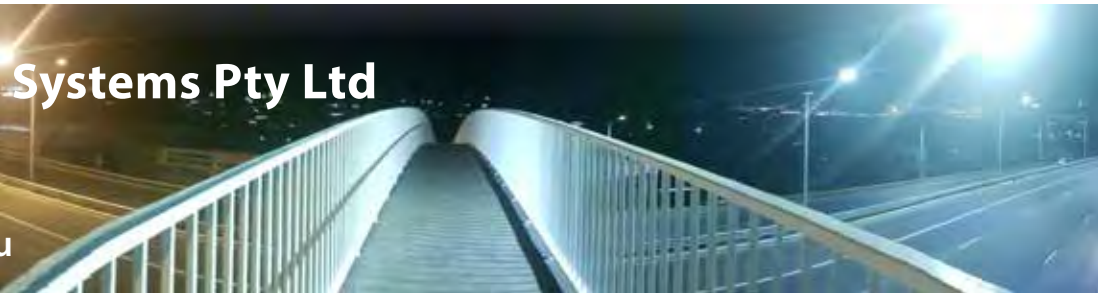
Before and After Installation - Hobart Tasmania
